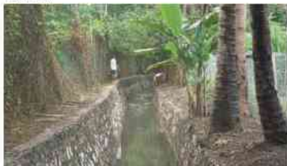
Opportunity for existing canals and waterways as an integrated "green-blue" landscape strategy.
