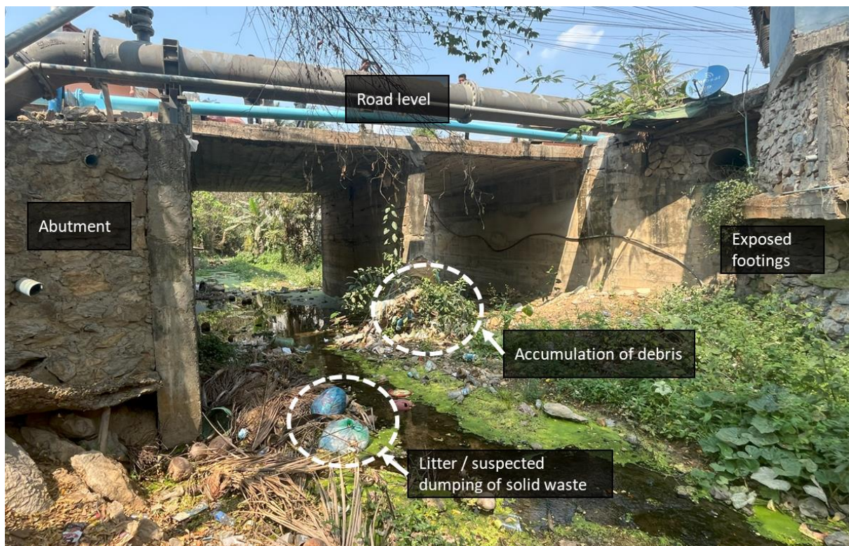
Figure 12. Huai Mao Bridge, Nasangvuey village (facing downstream)
