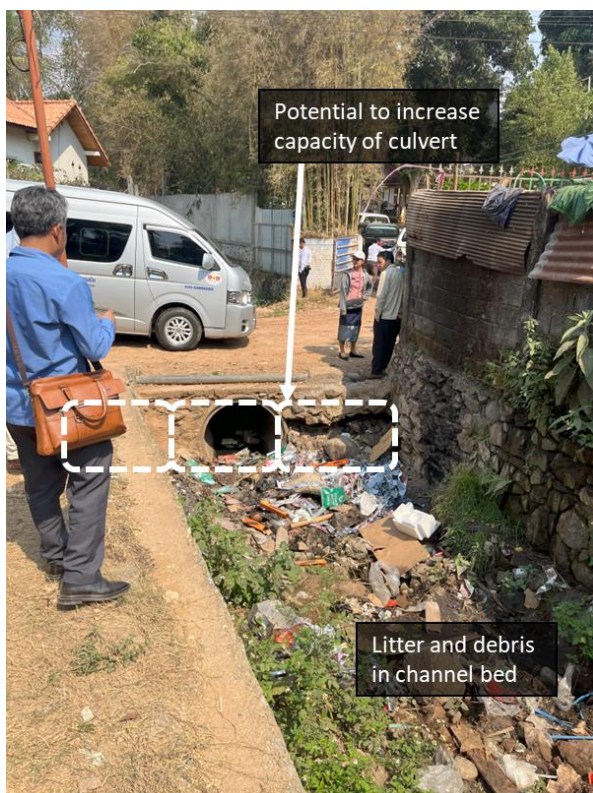
Figure 15. Road culvert (facing downstream)
