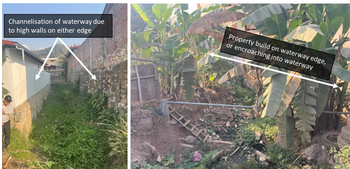
Figure 31. Examples of waterways impacted by encroachment and channelisation from adjacent buildings
