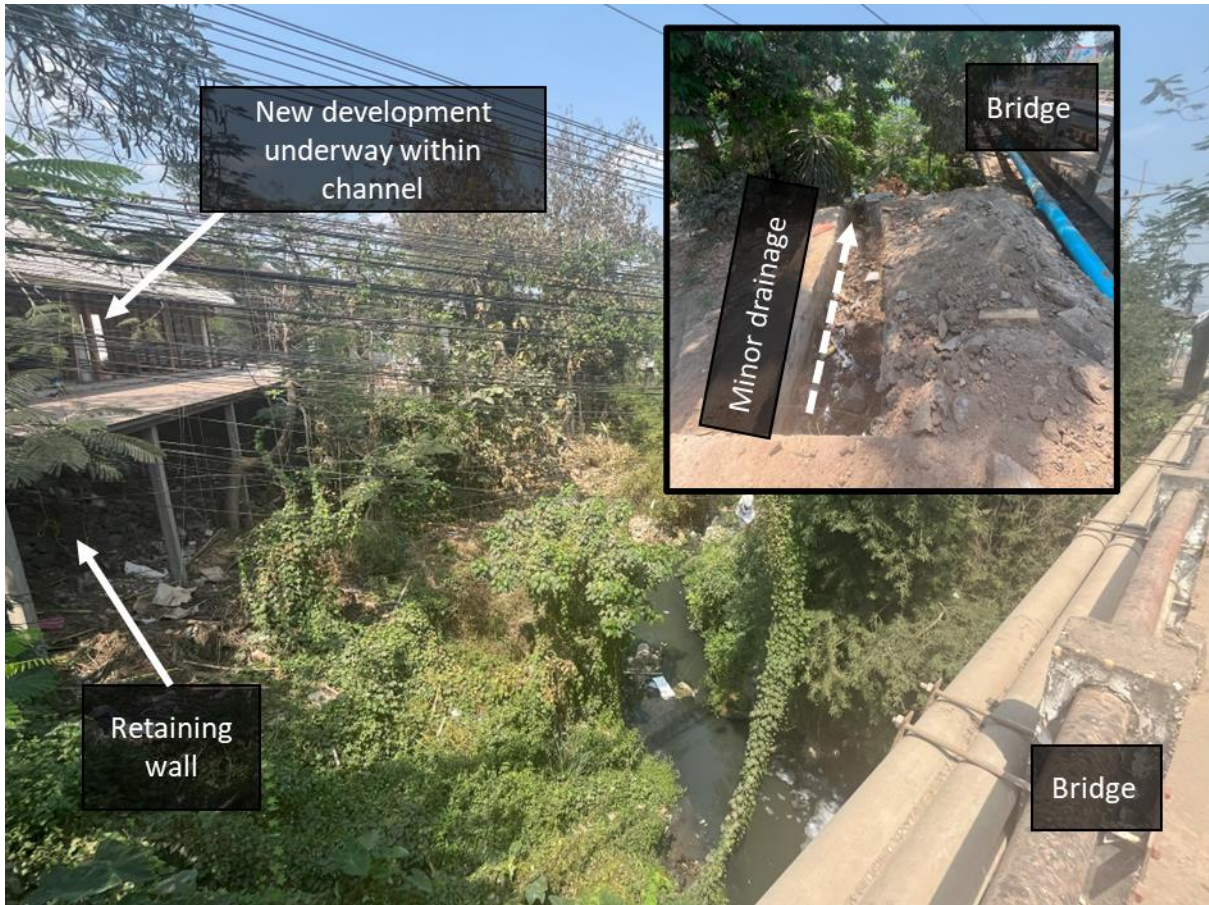
Figure 29. View toward of the Houay Hope River from the Houay Hope River bridge with an example of the minor drainage system at bridge/road level shown inset.
