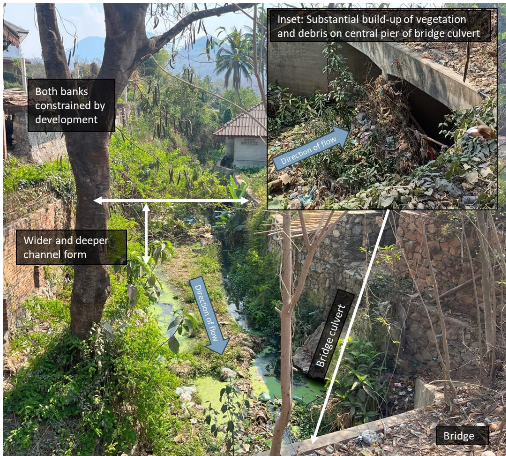
Figure 21. Road 12 Bridge (facing upstream)
