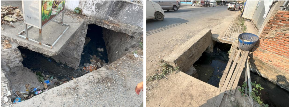
Figure 24. Examples of covered channels with perpendicular junctions
