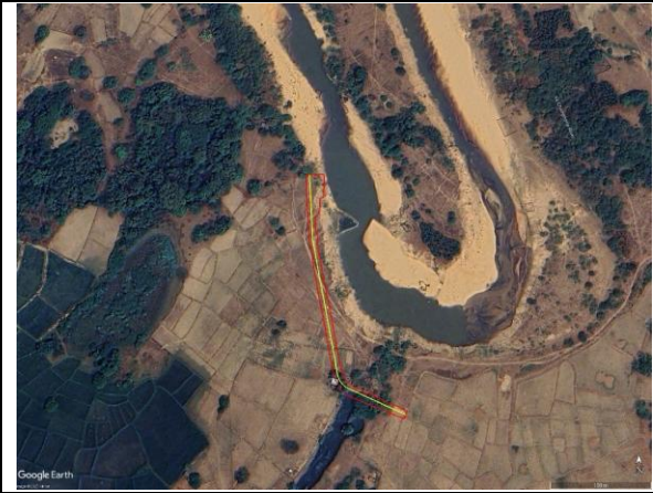
Flood protection levee in Phiaka Village, Champhone District
