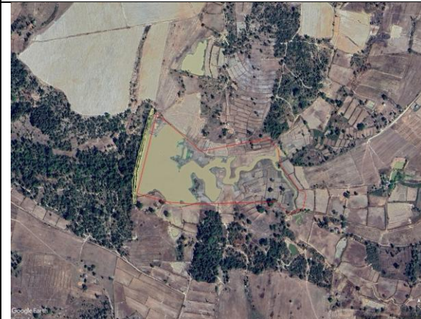
Upgrading 1 st community pond in Sivilay Village, Champhone District
