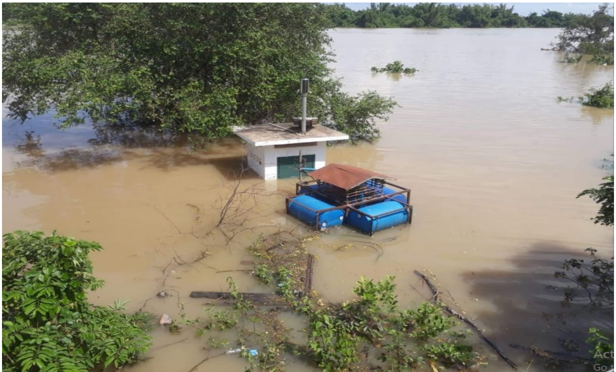
Figure 13. Flooding 2019 Xianghome station, Xonbouly district
